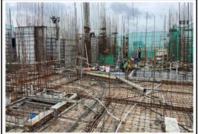
R10 LEVEL (16TH COLUMN R/F WIP) (Aluform)
