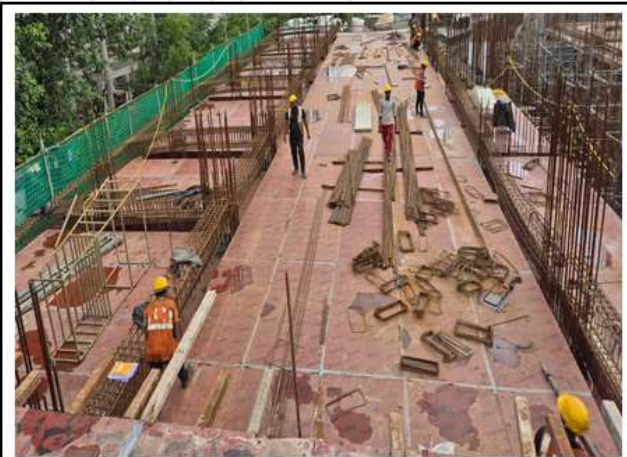
P1 LEVEL (3rd RCC SLAB) - (5.2 M)
