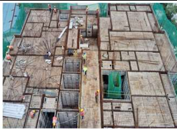
R08 LEVEL (14TH SLAB ) (Aluform)
