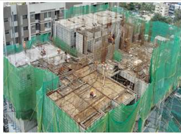
R10 LEVEL (16TH SLAB SHUTTERING WIP) (Aluform)
