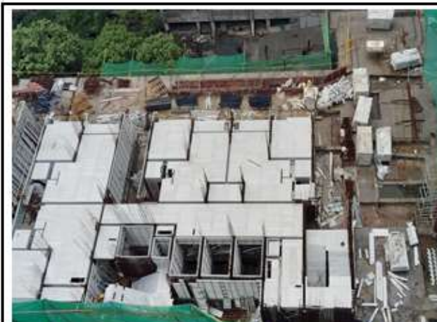
EL SLAB SHUTTERING WIP (8TH SLAB ) (3.05 M) ALUFORM
