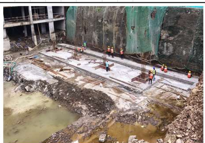
TOWER - B (RAFT & RETAINING WALL )
