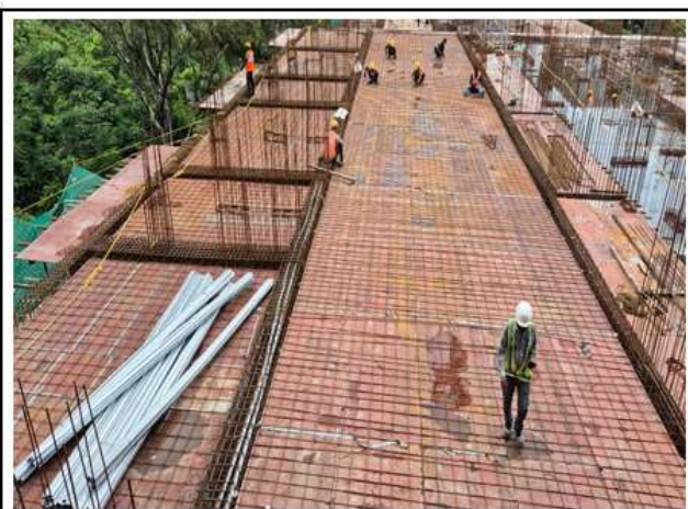
P2 LEVEL (4TH RCC SLAB SHUTTERING) - (3.0M)
