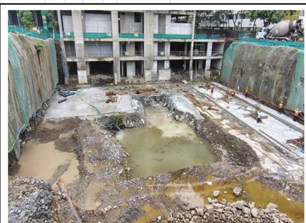
TOWER - B (PCC)
