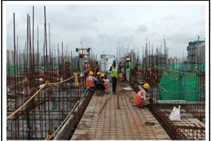
R08 LEVEL (14TH SLAB ) (Aluform)
