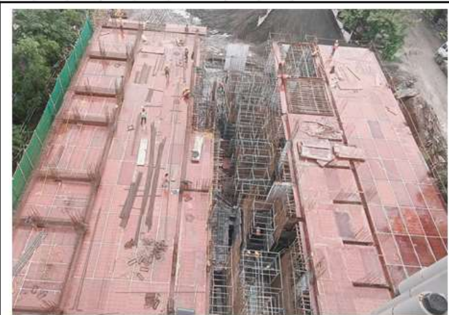
P1 LEVEL (3rd RCC COLUMN) - (5.2 M)
