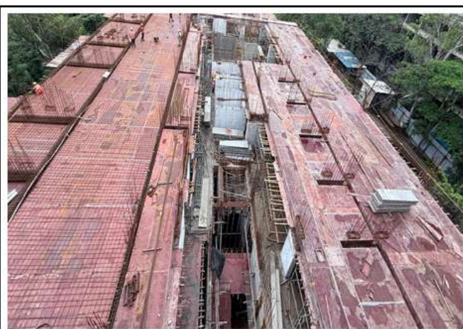
P2 LEVEL (4TH RCC SLAB SHUTTERING) - (3.0M)
