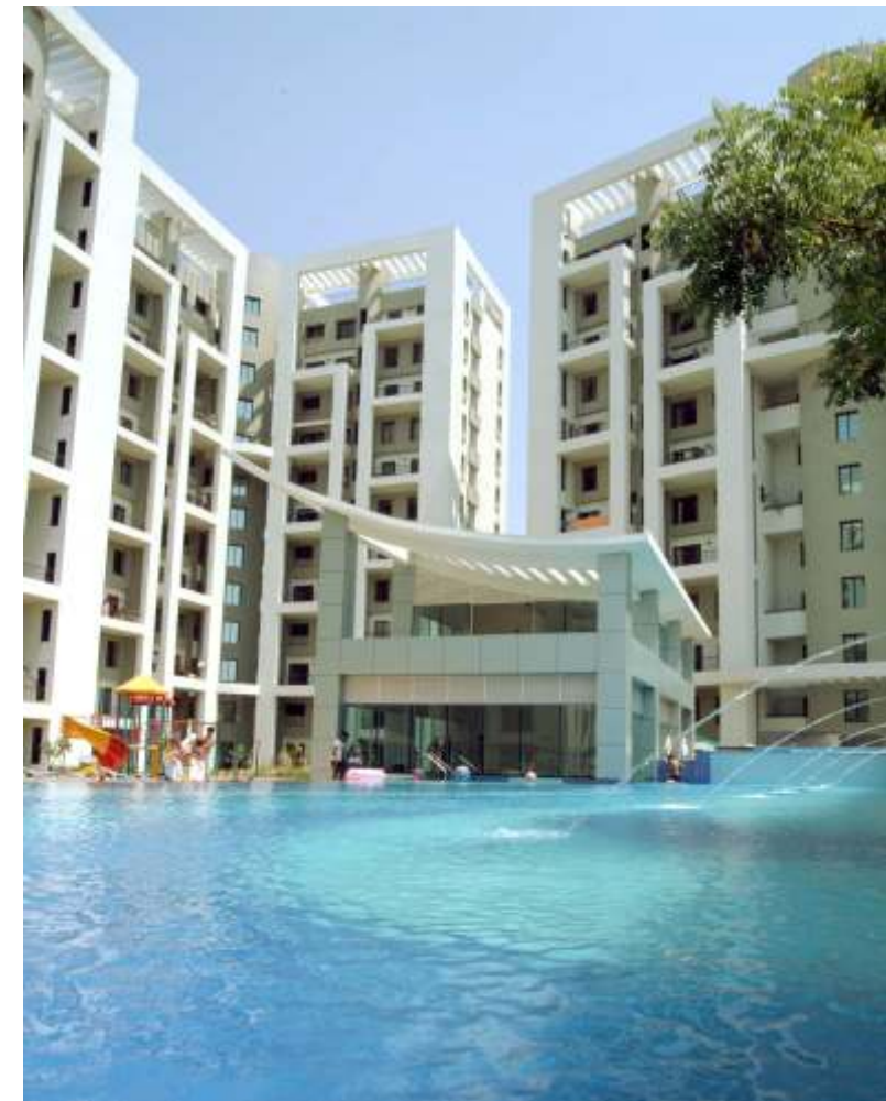
Rohan Tapovan, Pune
