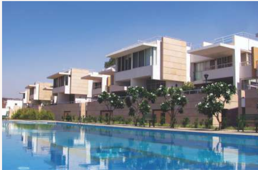
Rohan Madhuban, Bavdhan, Pune
